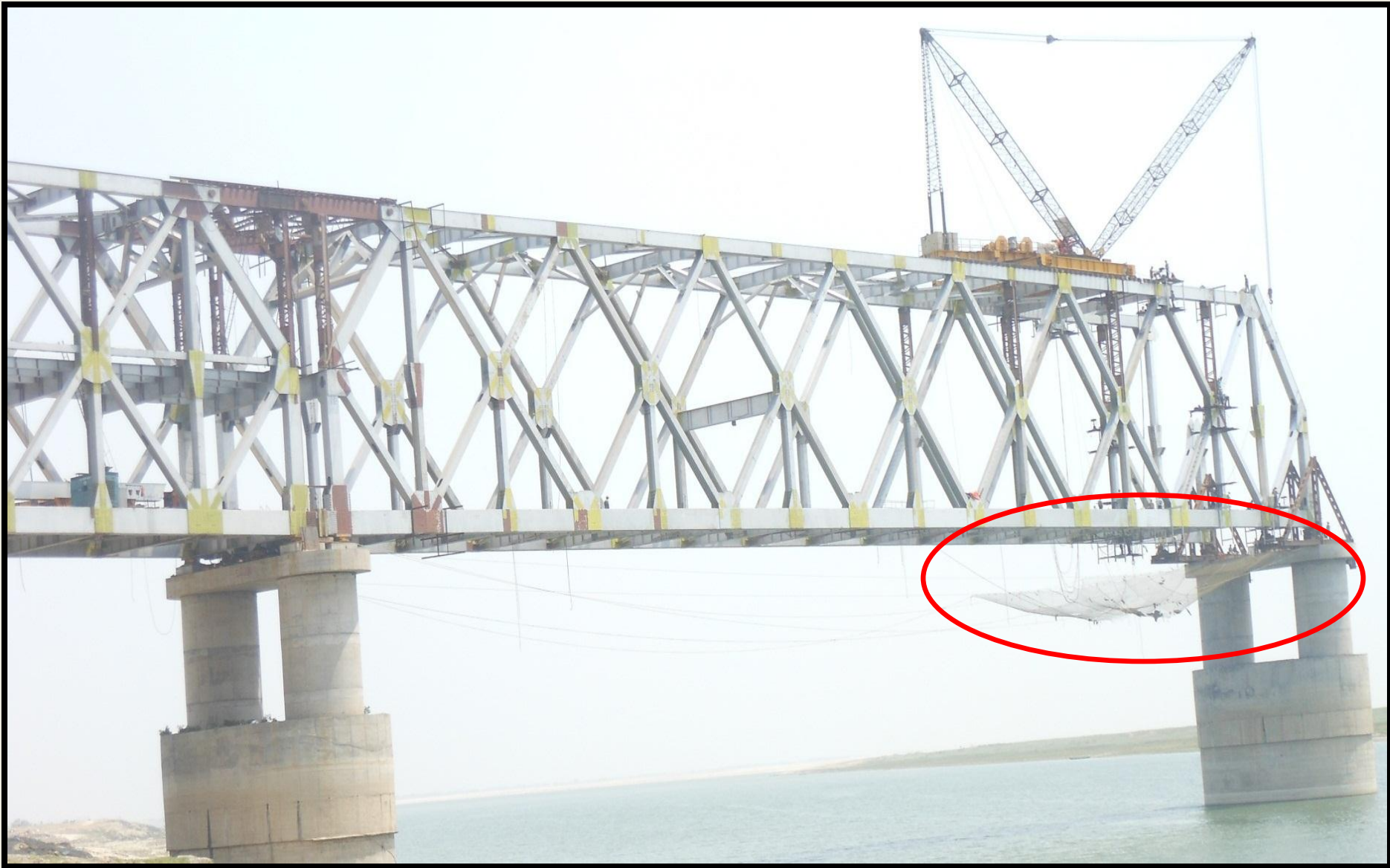
Safety Nets in use during the Cantilever Erection of Rail-cum-Road bridge in Munger, Bihar
