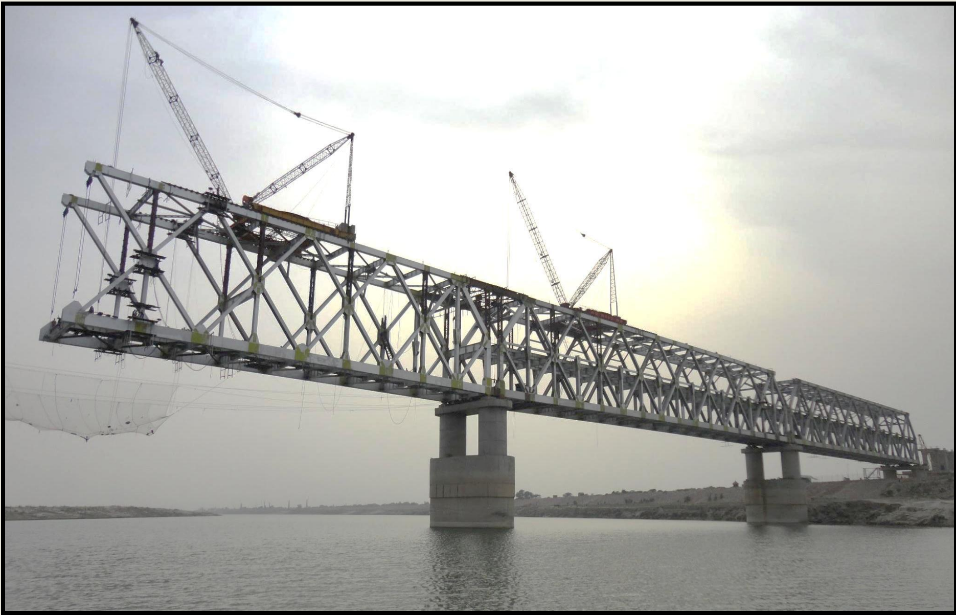
Longest span (125m) of cantilever erection of rail-cum-road bridge at Munger, Bihar
