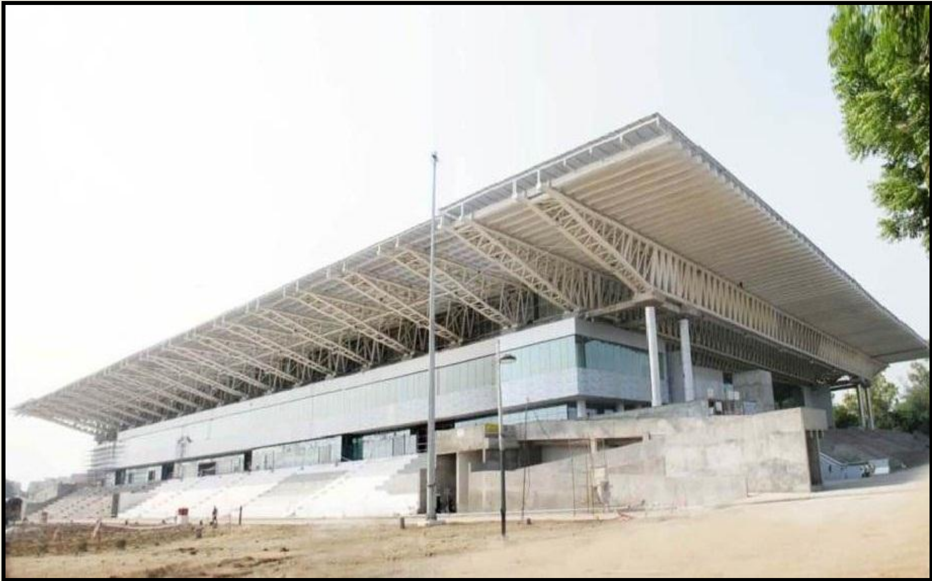
Longest Steel Truss Of 107m Span For Thyagraja Netball Stadium For Commonwealth Games 2010, Delhi
