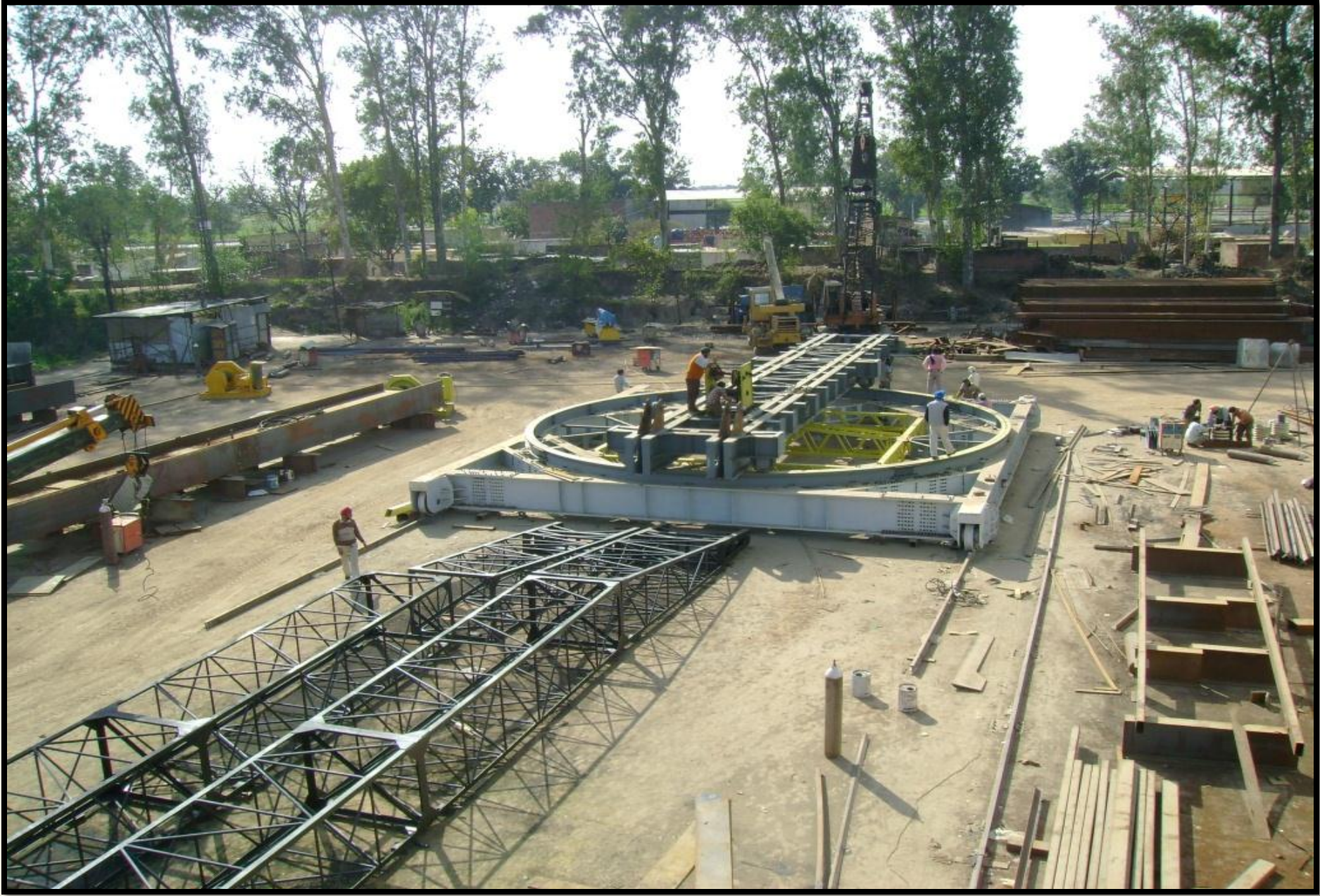
Fabrication of Erection Crane for Munger Site
