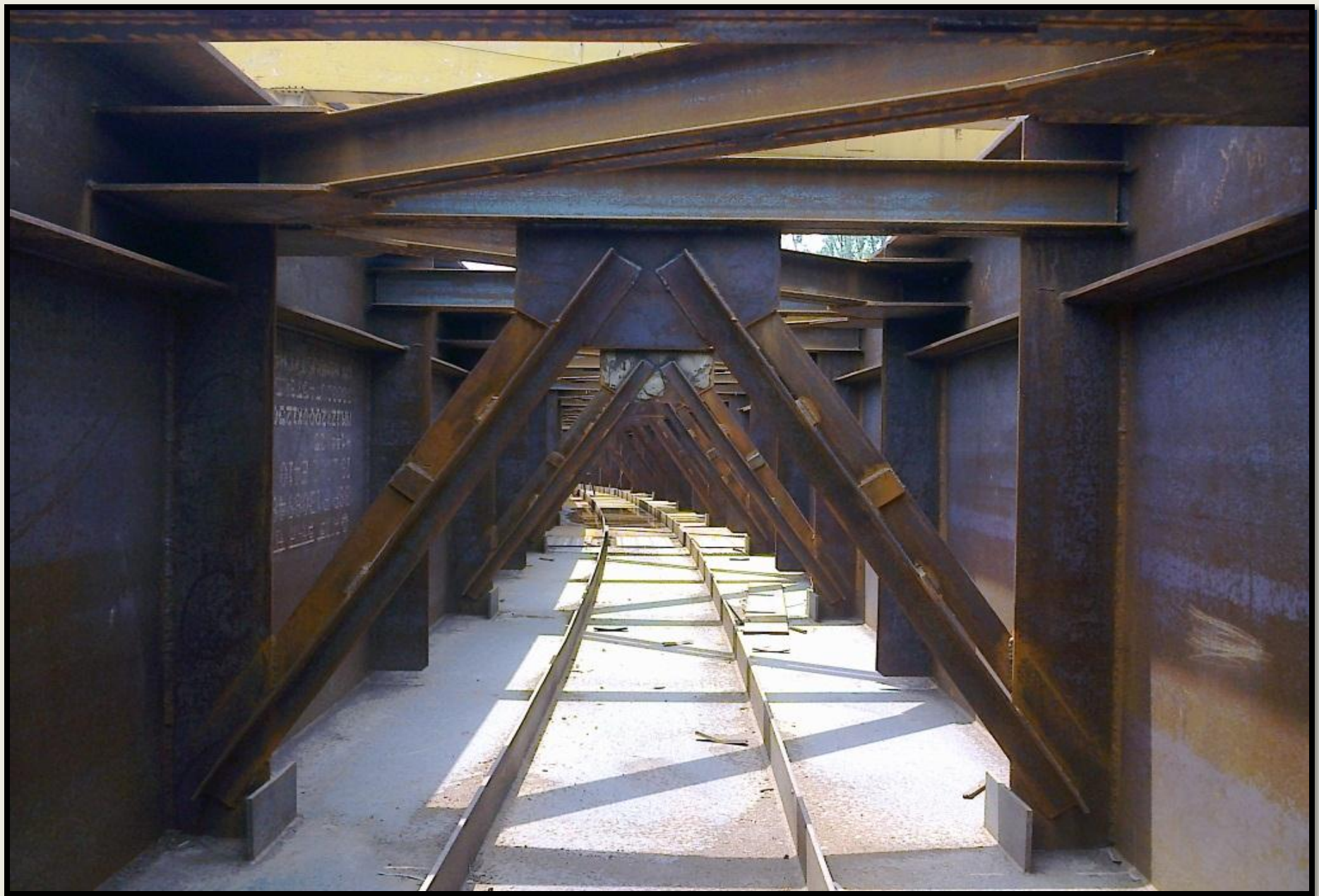
Internal View of the Fabricated Box type Girder Assembly
