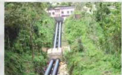
Panniar HEP Rehabilitation, Kerala
