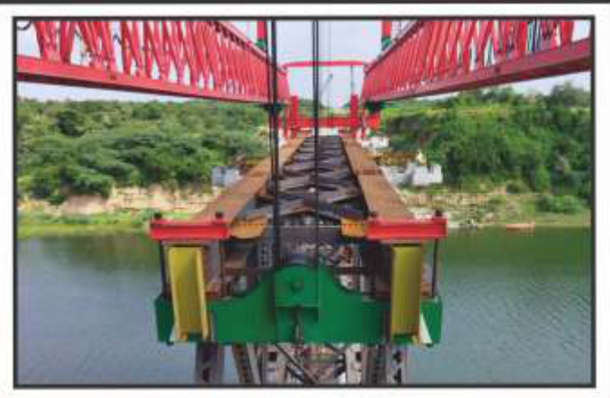
DFCC Underslung Truss Bridge, Baroda
