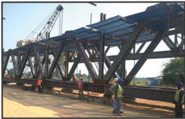
Site Assembly of Underslung Truss Bridge, Ahmedabad
