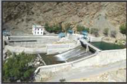
9 MW Dah, HEP, Ladakh
