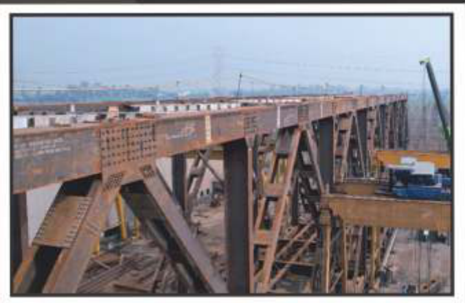
Trial Assembly, Mokama Railway Bridge at our Fabrication Facility
