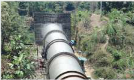
UHL-Stage-III-(100MW) HEP, Himachal Pradesh
