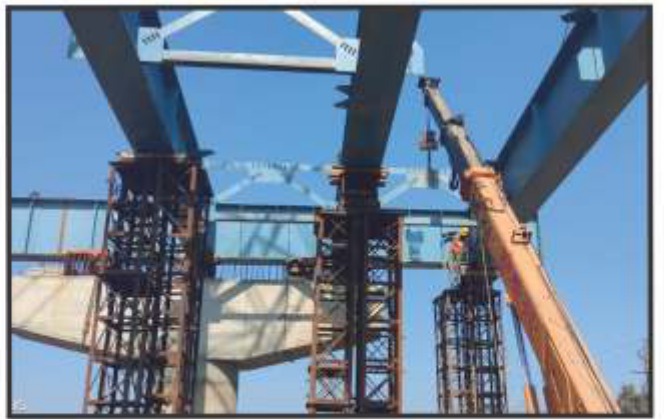
Erection of Plate Girder, Panipat
